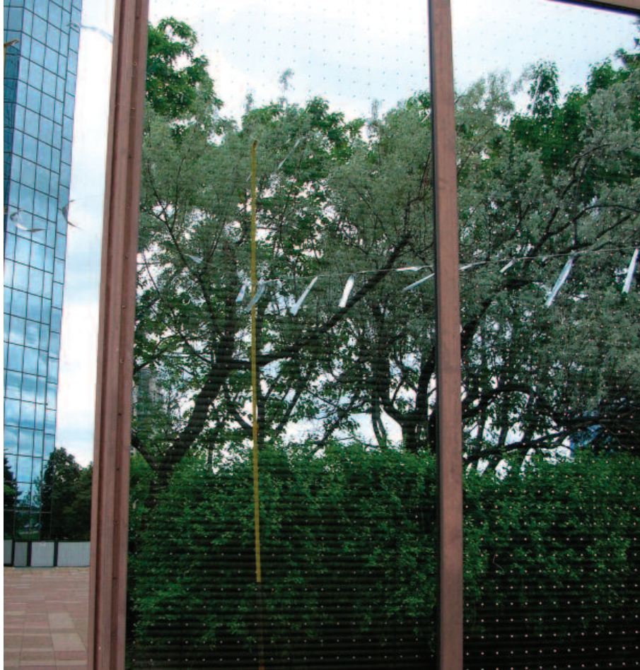
Glass treated with properly spaced visual patterns is proving to greatly reduce daytime collisions.
