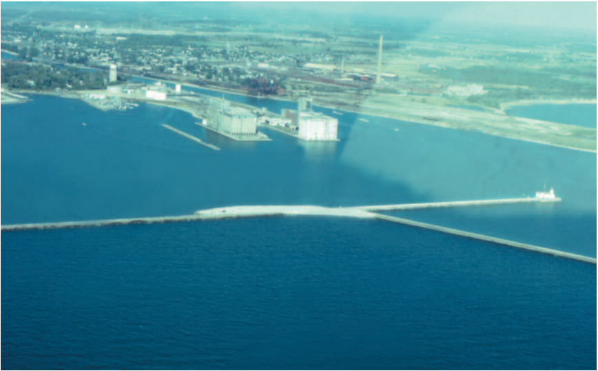
Figure 3. An aerial photograph (facing north) of the Port Colborne Breakwall, Lake Erie in the early 1980s. The rockpile is the white area on the north side of the breakwall, at the junction of the southern and east-west arms. Photo by Ralph Morris.
