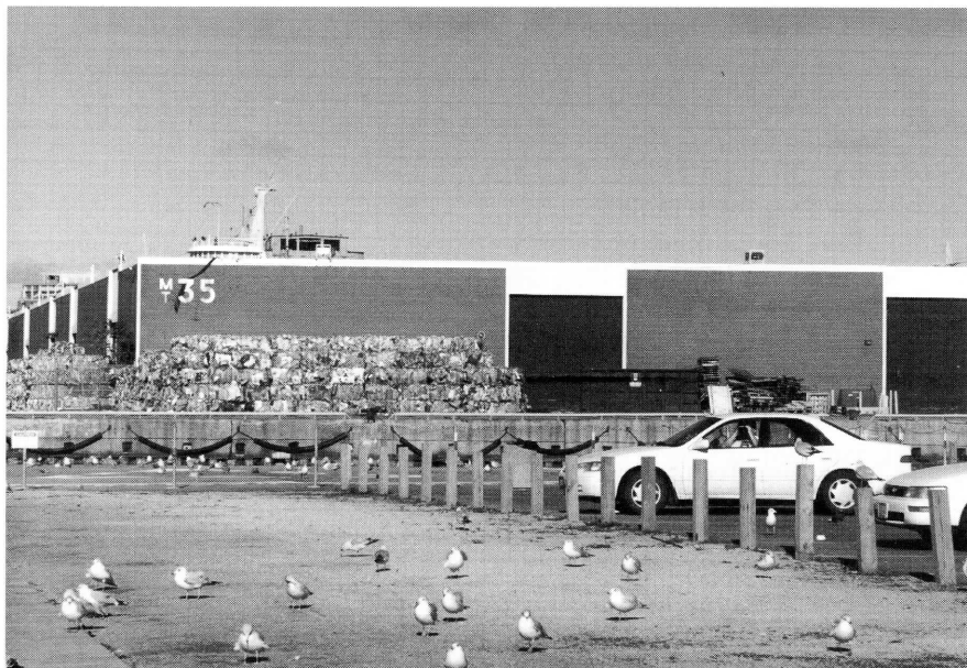
Figure 1: Flat-roofed building at Toronto Harbour utilized by Caspian Terns as a night roost site. Photo by Jean Iron.
